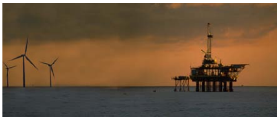
Ageing Management should be addressed from the design phase and not when the design life is due to expire.
