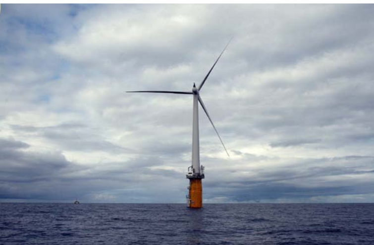
Hywind is the very first full scale floating wind turbine installed offshore. A scale model of the turbine was tested in the MARINTEK Ocean Basin for proof of concept. Photo: Trude Refsahl / Statoil
